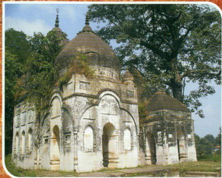
Ichak Group of Temple, Ichak, Hazaribagh.
